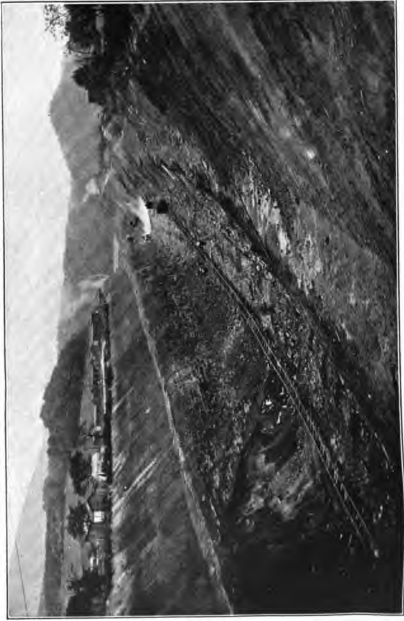
PLATE X.—Deep Cut near Pawpaw on Magnolia-Pawpaw Low Grade Line of Baltimore and Ohio Railroad, showing Catskill Shales and Sandstones with Overlying 25 Feet of Alluvium.
